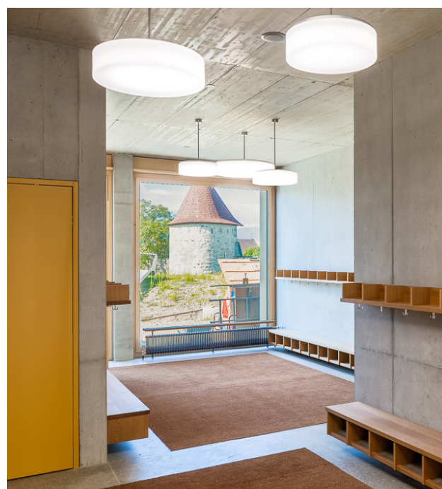
SPIN pendant luminaires of different sizes are arranged at various heights in the changing rooms.
